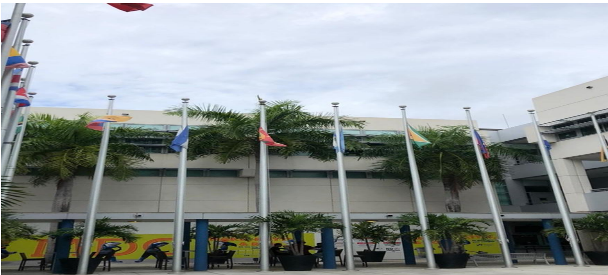
Eduardo J. Padron Campus, view of Building 1 from flag Courtyard.
